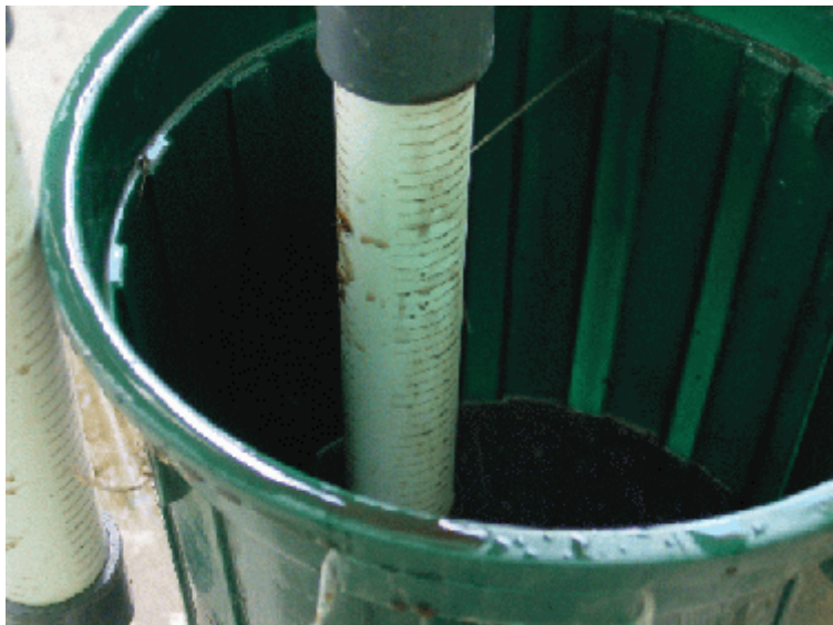
Figure 9 Closeup of one of the pipes following partial manure sealing
