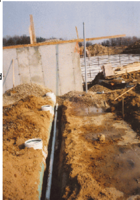
Figure 5 Sampling pipe in trench next to pull plug transfer pipe
